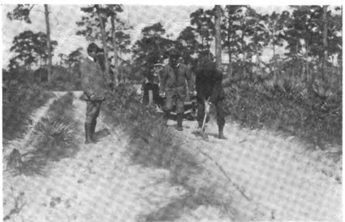
REMOVING A STUMP THAT BLOCKED THE WAY.
